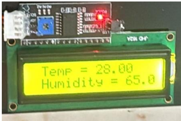
Fig 2: Temperature and Humidity Levels
