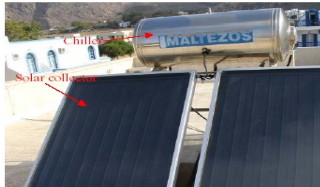
Fig: Flat-plate solar-powered single-effect absorption cooling system.
